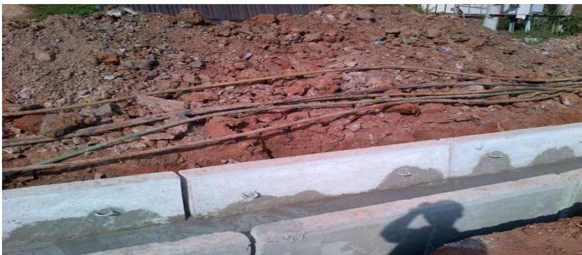
Figure 1.1 Uprooted Optic fibre cable along a major road in Nigeria.
