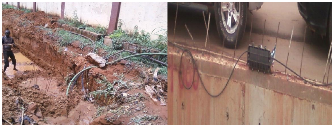
Fig 2.1 Damages on fibre optics cable
