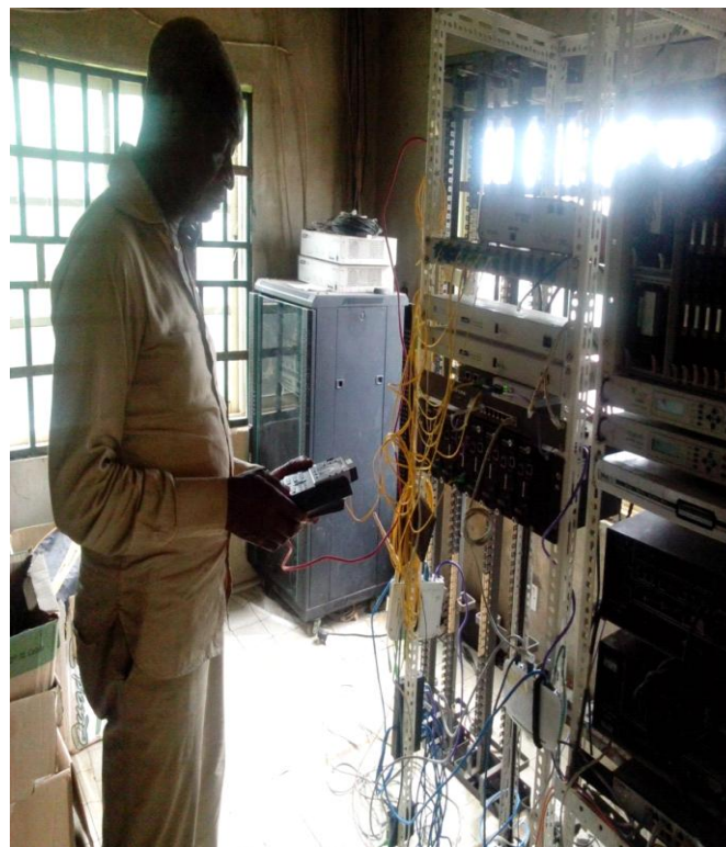
Fig 2.12 Power budget test
