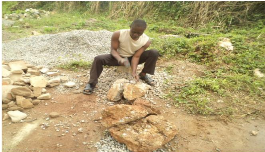
Plate 2.1c: Showing the process of breaking the demolished concrete
