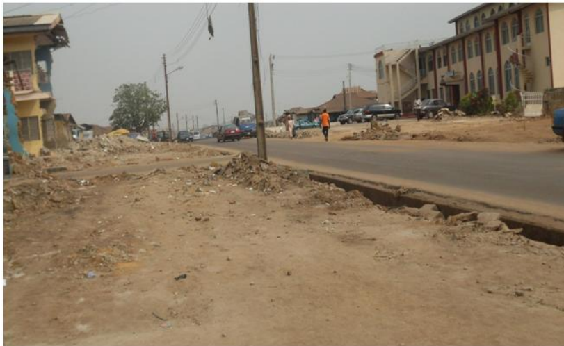
Plate 2.1a: Arakale Street Undergoing Building Demolishing Due to Road Dualization.
