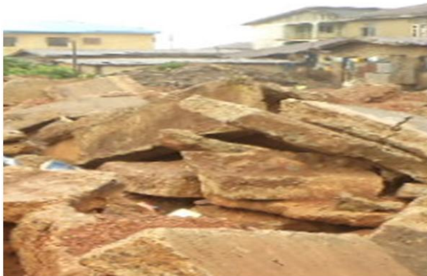
Plate 2.1b: Demolished Concrete Materials piled-up at the Site from which the sample used was taken.
