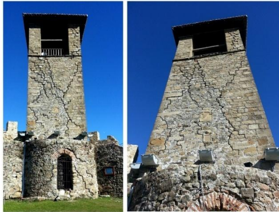
Figure 4. Structural cracks found on the main façade.
