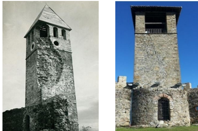
Figure 1. Clock tower: the past (a) and present condition (b)
