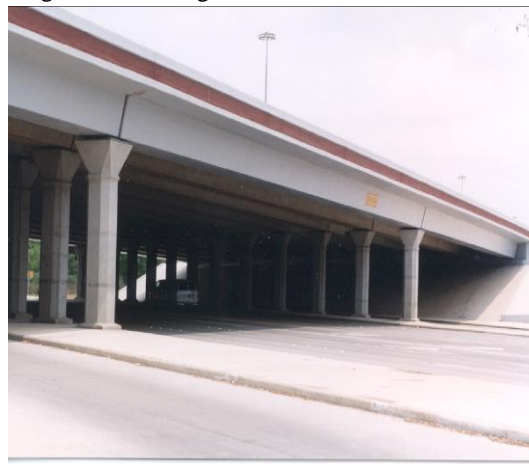
Fig.2 HPC bridge in Texas
