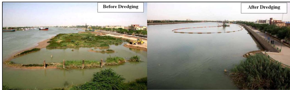
Figure 22: The impact of dredging operations in order to Karun River training in the Khorramshahr city
