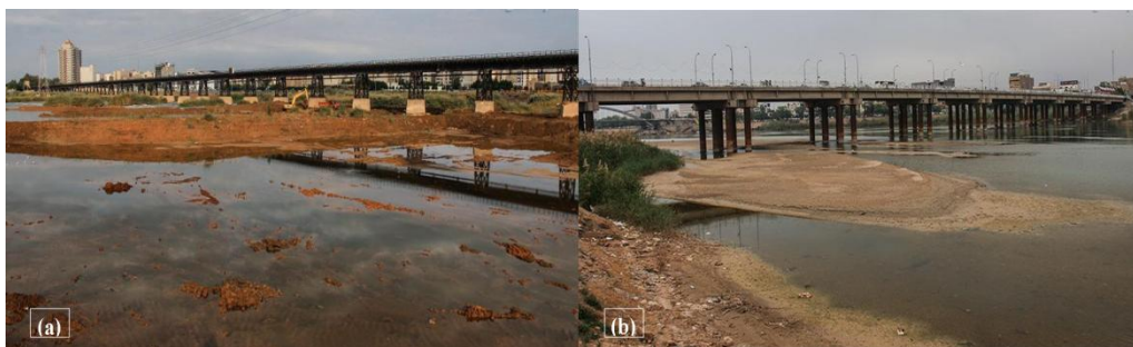
Figure 20: View of the islands formed by the river sedimentation at the downstream; a Siah bridge and b Naderi bridge
