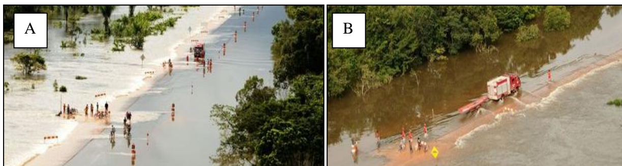
Figure 16. A. BR-432 flooded with traffic stopped. B. BR-174 with traffic stopped in the city of Caracaraí, RR. Source: A Crítica, 2011.
