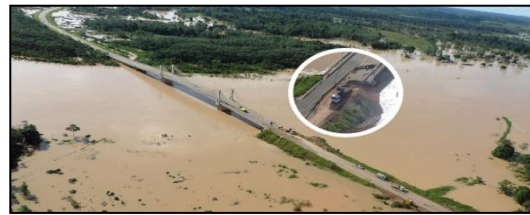
Figure 15. Bridge over the River Tarauacá (AC) with damage to its structure. Source: DNIT, 2014.
