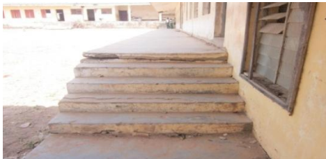
(A) Stairs Along Corridors And To Classrooms F.G.C) Minna
