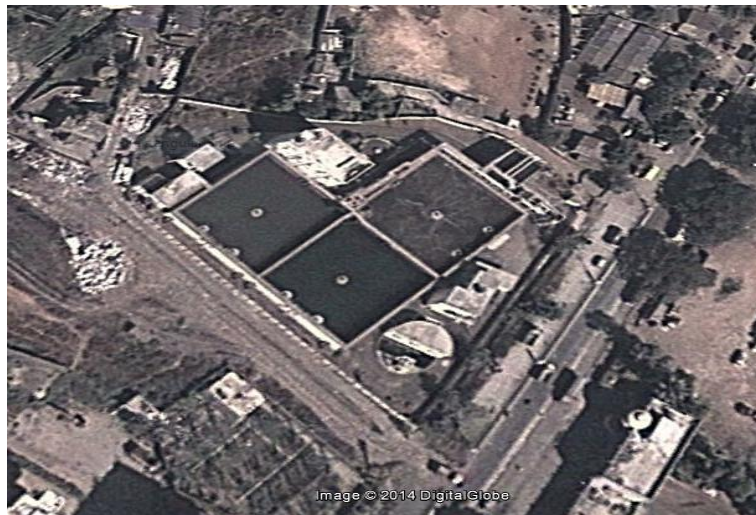
Figure 1: Google Earth Image of the Treatment Plant
