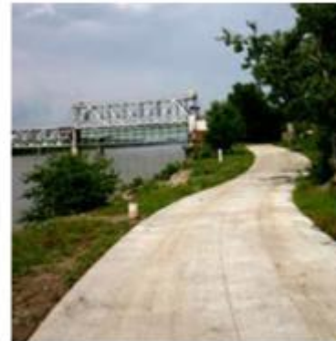
Photo 8: Road along the river side
