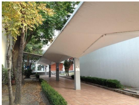
Figure 3. Corridor covered by a concrete shell, University Campus, BUAP (2013).
