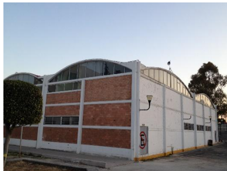
Figure 2. Lab building, Engineering Faculty, BUAP (2013).
