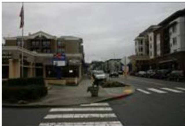
Figure 13. Double ramps align with crosswalks directs pedestrians into traffic [1].
