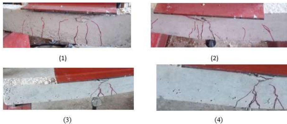
Fig. 4. Crack Pattern of test specimen: (1) Type-MC, (2) Type-M1, (3) Type-M2, and (4) Type-M3
