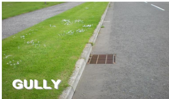
Fig 4: Gully design installation by the kerb on a road side
