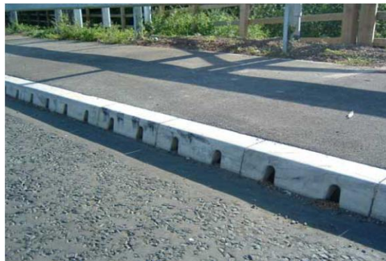
Fig 3: Drainage and kerb combination design example
