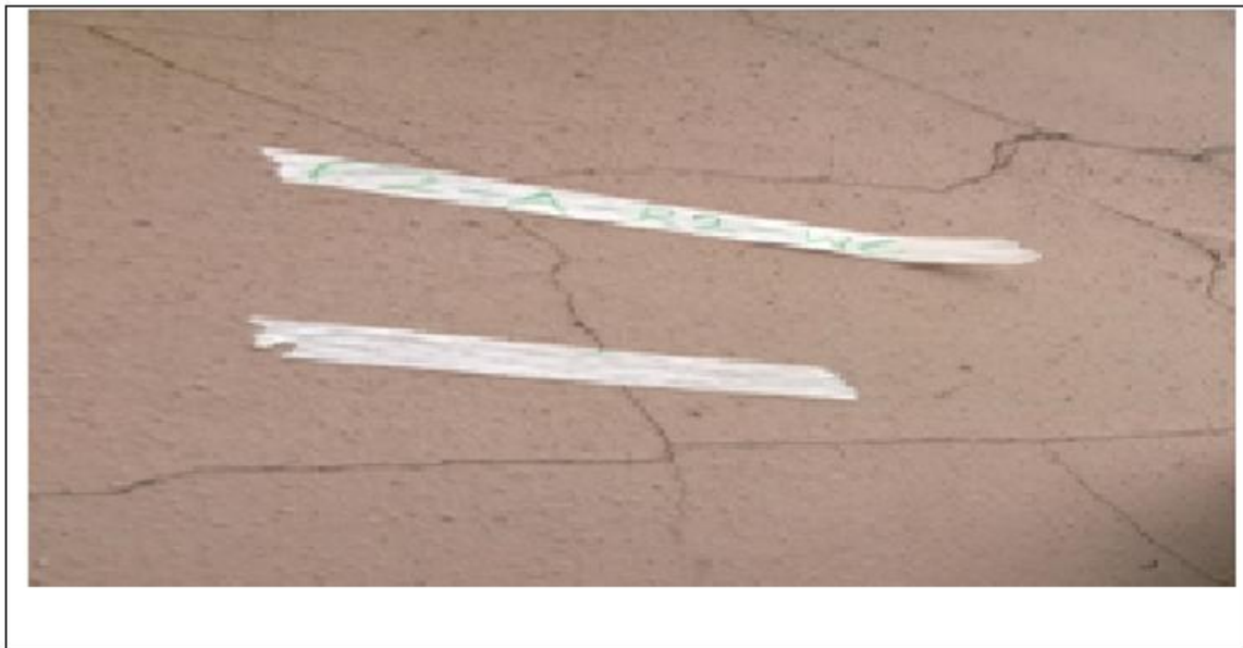
Plate 2. Picture of random cracks due to drying shrinkage
