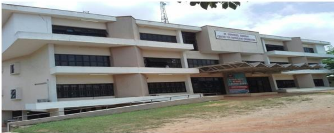
Plate 1. Front view of the building
