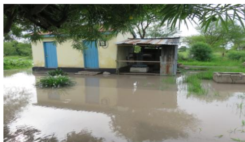
Figure 2: Pump house at the intake flooded with surface runoff
