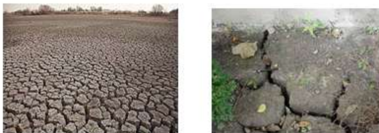
Fig 2. Views of expansive soil with Polygonal pattern of surface cracks in the dry season.
