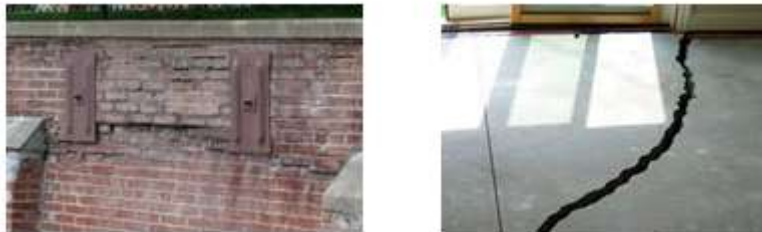
Fig 1. Views of cracks in exterior walls as a result of upward soil expansion
