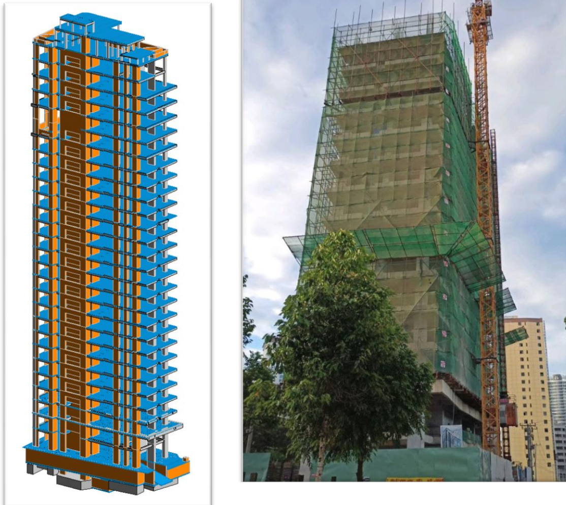
Fig. 10. The Modeling Realistic in Revit with real Construction Site
