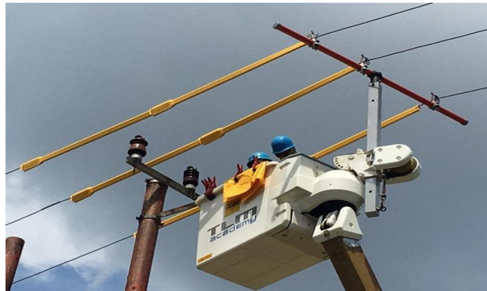
Fig.2. Installation of pedestal isolators in a stressed state Using the Direct Touch Method (source: www.pdkb.id)
