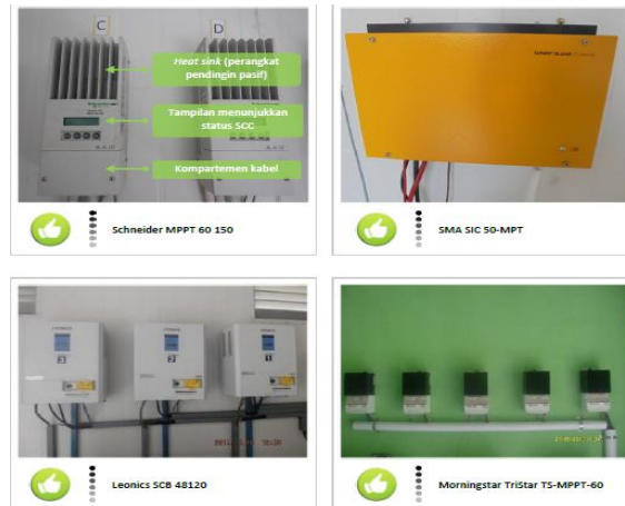
Figure 3. Solar charge controller (SCC)
