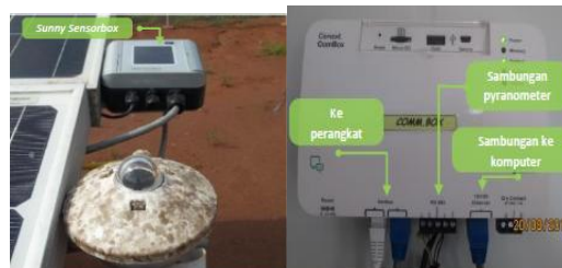
Figure 8. Monitoring System and Pyranometer
