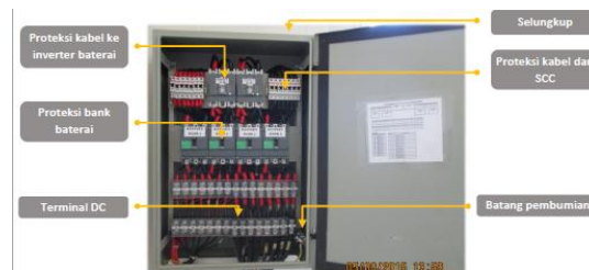
Figure 4. DC Distibution Panel
