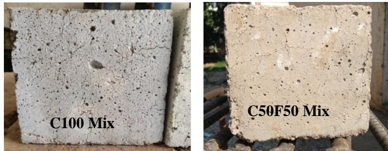
Figure 2: Cracks observed at 600°C
