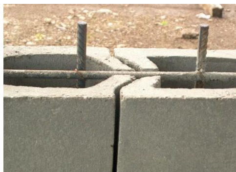
Figure 3. Interlocking blocks with vertical and horizontal rebar
