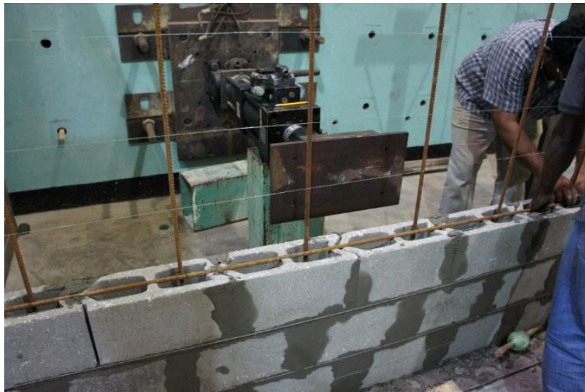
Figure 4. Wall section under construction with vertical and horizontal rebar
