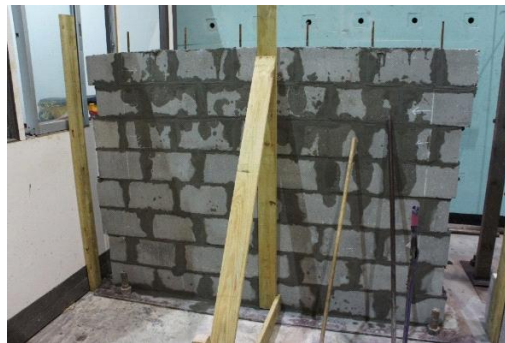
Figure 2. Completed interlocking block wall section with vertical rebar
