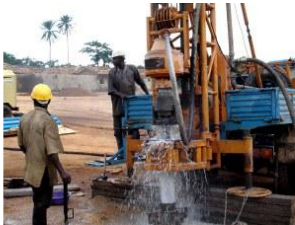
Figure 3: Typical borehole drilling showing water flow
