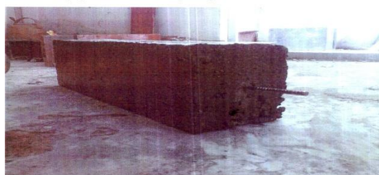
FIGURE:- Beam with sulphur coated steel bar
