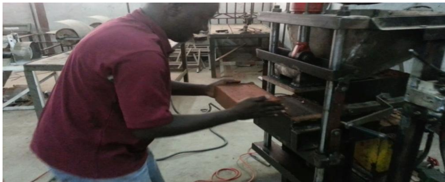
Figure 2.5 Compressed Soil Block lifted to curing yard
