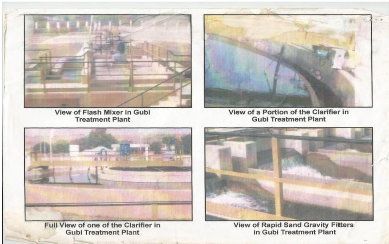
Figure2. View of Gubi dam Treatment Plant
