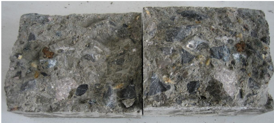
Fig. 3. Recycled Aggregate Concrete Failure by way of Tensile
