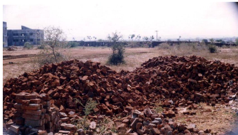
Fig 2 Improper stackig of brick
