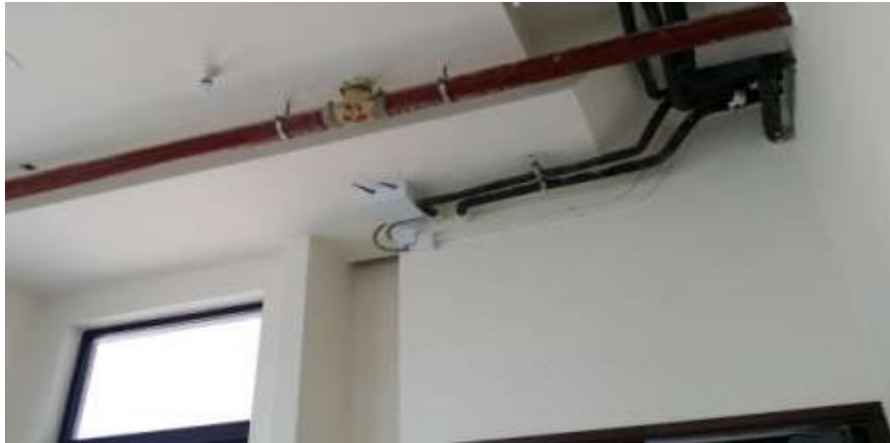
Figure 2.3.5 Equipment Box for the home automation module
