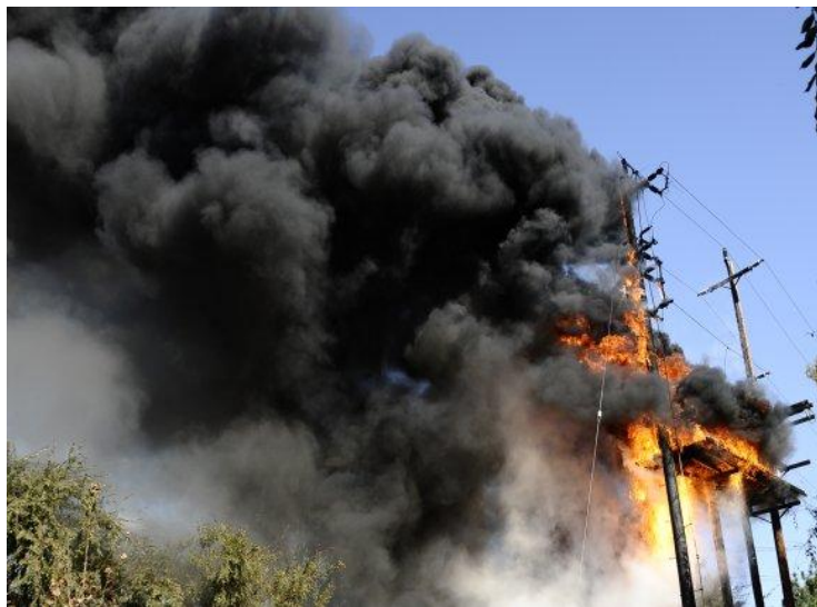
Figure (2): A Three Phase Pole Mounted Distribution Transformer Blasts
