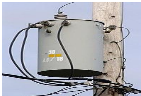
Figure (1): A Three Phase Pole Mounted Distribution Transformer
