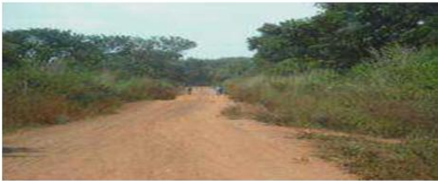
Picture 1: Partially-Engineered Feeder Road
