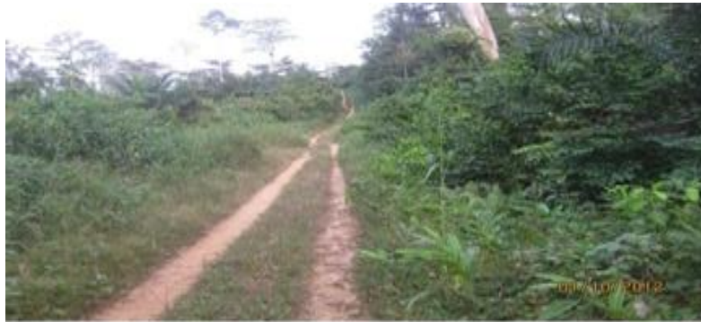
Picture 3: Un-Engineered Feeder Road
