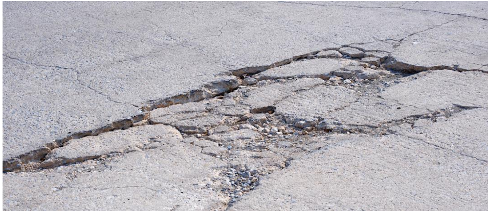
Fig. 1. Freeze-Thaw Damage to Concrete
