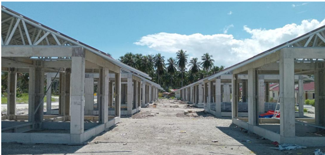
Figure 2. Practical working method in RISHA construction by connecting concrete panels using bolts
