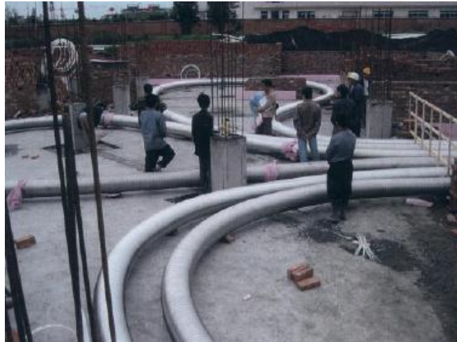
Fig.7. ISOMAX "pipe in a pipe" countercurrent device [2], [27], [28]
