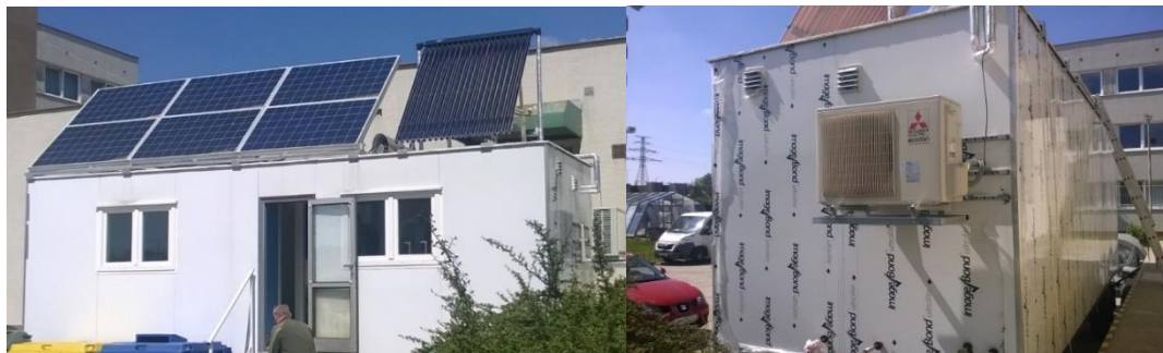
Fig.15. Mobile laboratory - optimizer and simulator of compact heating / cooling units [6, 15]
