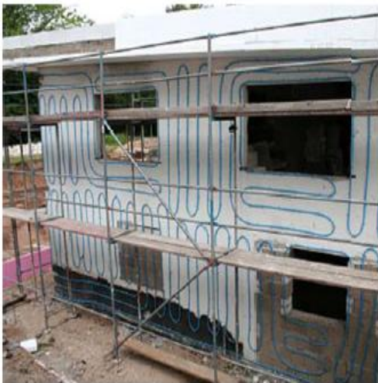
Fig.6. Two-pipe wall energy system ISOMAX in the sense of patent SK 284 751 [2], [12], [27], [28]
