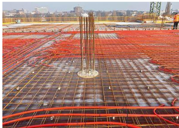
Fig.2. Thermal activate building structures [34]
