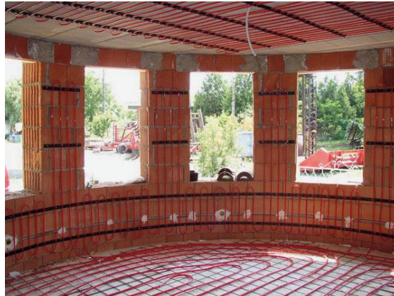
Fig.1. Large area low temperature heating and high temperature cooling systems [34]
